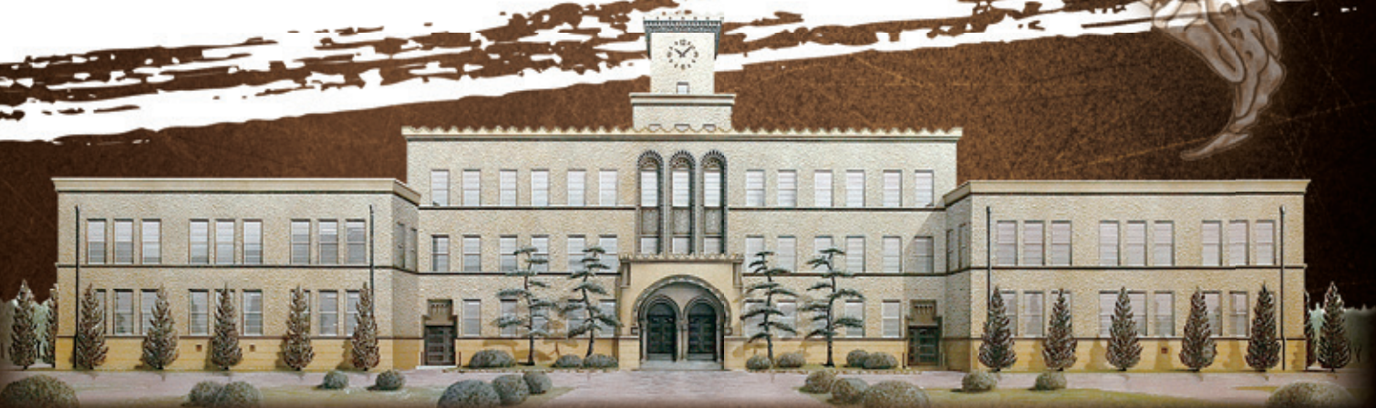
大阪医科大学 旧本館 The Former Main Building of Osaka Medical College
